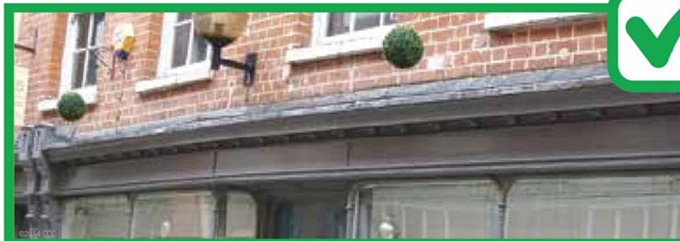
A moulded shopfront cornice with dentilated detail on the underside.
